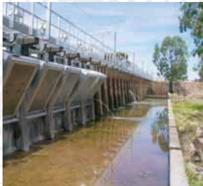
> Horsham Weir, Wimmera region, Vic (Wimmera CMA)
