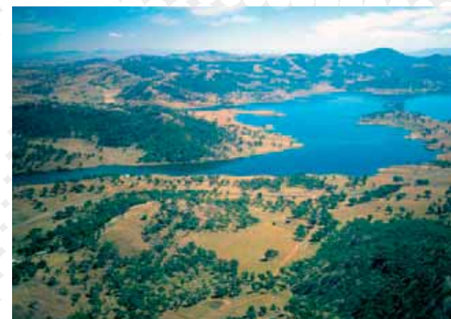
> Chaffey Dam, Namoi region, NSW (CSIRO)
