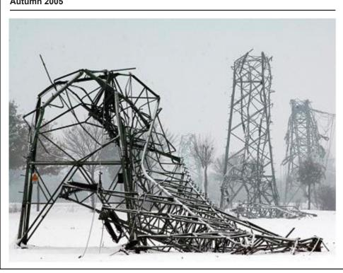
Figure 3.2. Extreme Ice and Snow Loads on Pylons Near Münster, Germany, in Autumn 2005
