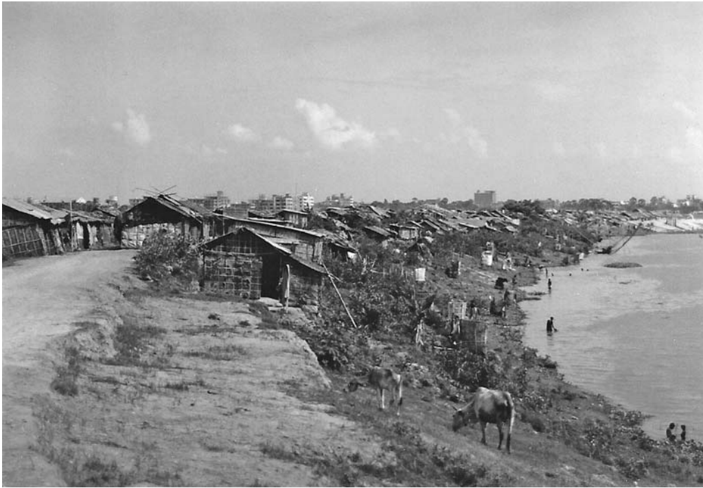
Photo 3.17: Multipurpose embankment with erosion. Source: Alan Bird
