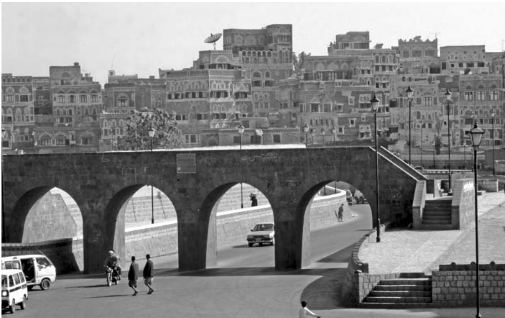
Photo 3.7: Roadway/flood channel Yemen. Source: Bill Lyons/World Bank
