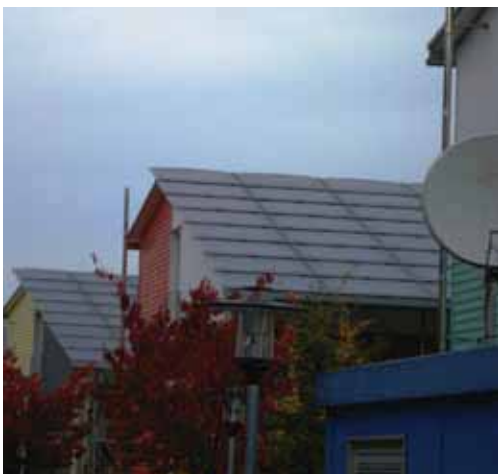
Solar PV panels on the rooftops of the "energy plus" houses © Gabriela Weber de Morais, 2009
