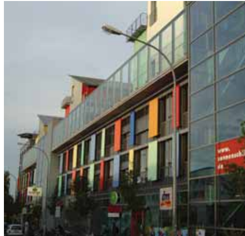
The "solar ship" mixed use building in Vauban's solar settlement © Gabriela Weber de Morais, 2009
