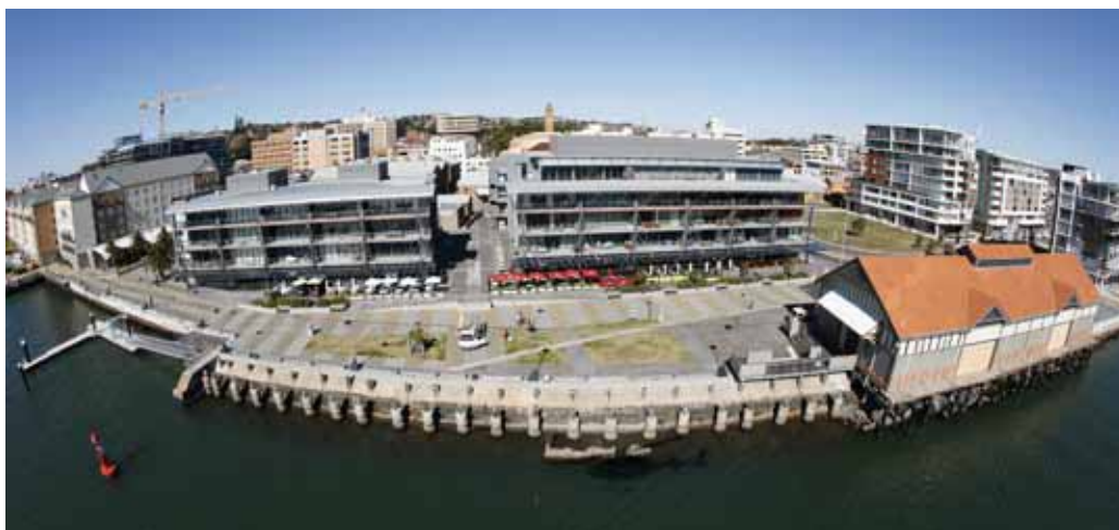
Boardwalk and Maritime Centre at the Honeysuckle development © Hunter Development Corporation, 2008
