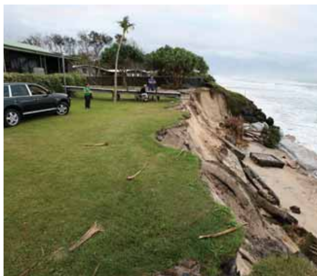
Severe beach erosion along Belongil Beach at Byron Bay, May 2009, where many metres of sand were washed away.
