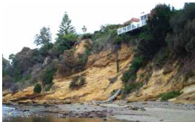
House sited on a coastal cliff that is prone to slumping.
