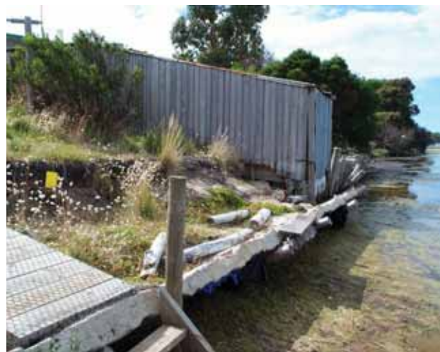
Eroding soft rock shore (clayey gravels) at Anson's Bay, north east Tasmania. The photo (2002) shows a poorly constructed ‘coastal defence’ that is collapsing because of undermining of the shore in front.
