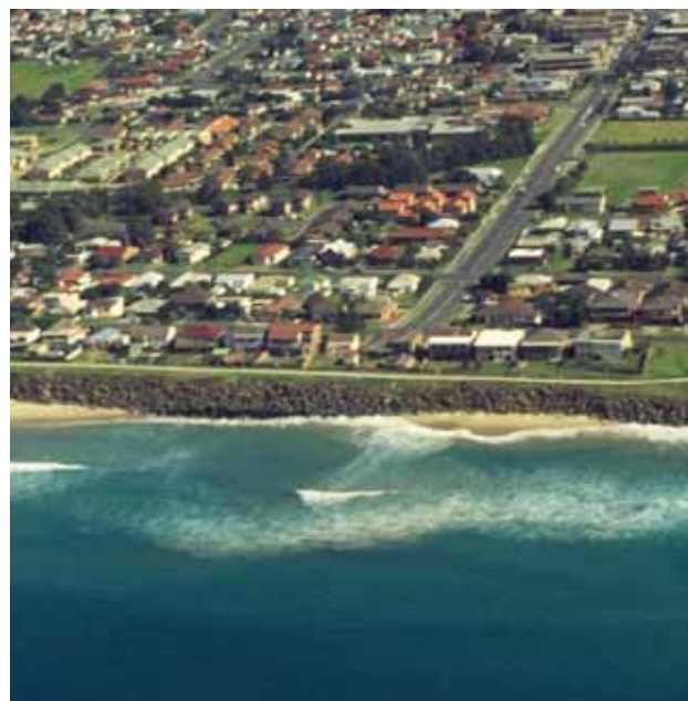
The surf club had to close and move when the seawall was built at Warilla.
