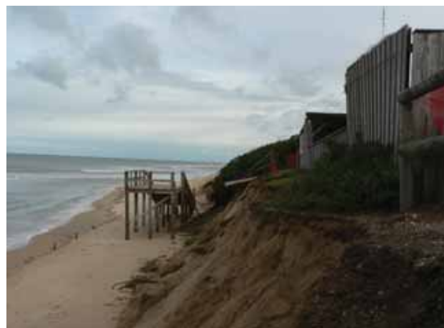
Erosion along Ninety Mile Beach.
