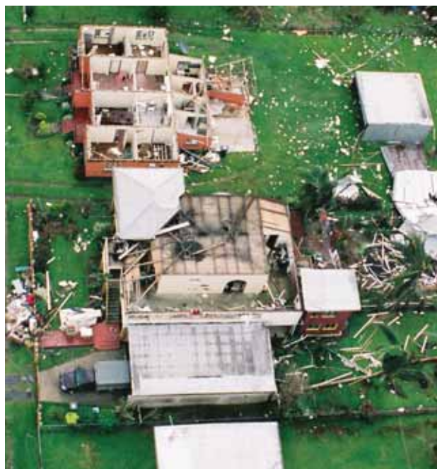
Damage to houses in Innisfail, Queensland caused by Tropical Cyclone Larry.
