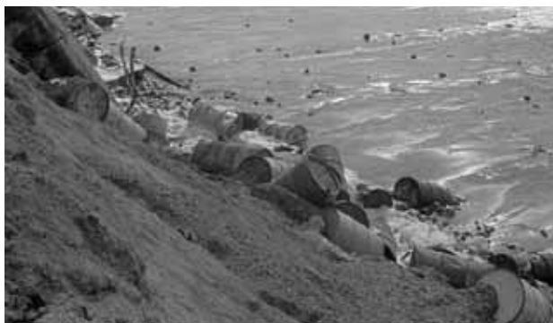
Forty-four gallon drums filled with concrete to prevent further beach erosion on the Gold Coast, 1967.
