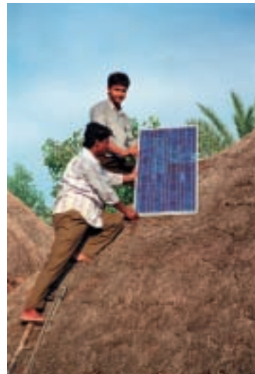
Installing solar panels as part of a new service module
