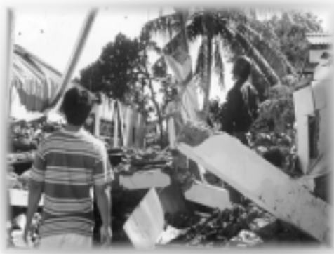
Most damage to residential housing was mainly to nonengineered houses and new “modernized” masonry houses. Aside from the paradigm shift towards modern life-style values and the poor quality of the design and construction
