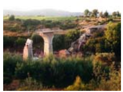
27 February Earthquake, tsunami: Chile Overall losses: US$ 30,000m Insured losses: US$ 8,000m Fatalities: 520
