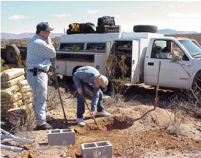
Installation of SCAN station in Arizona
