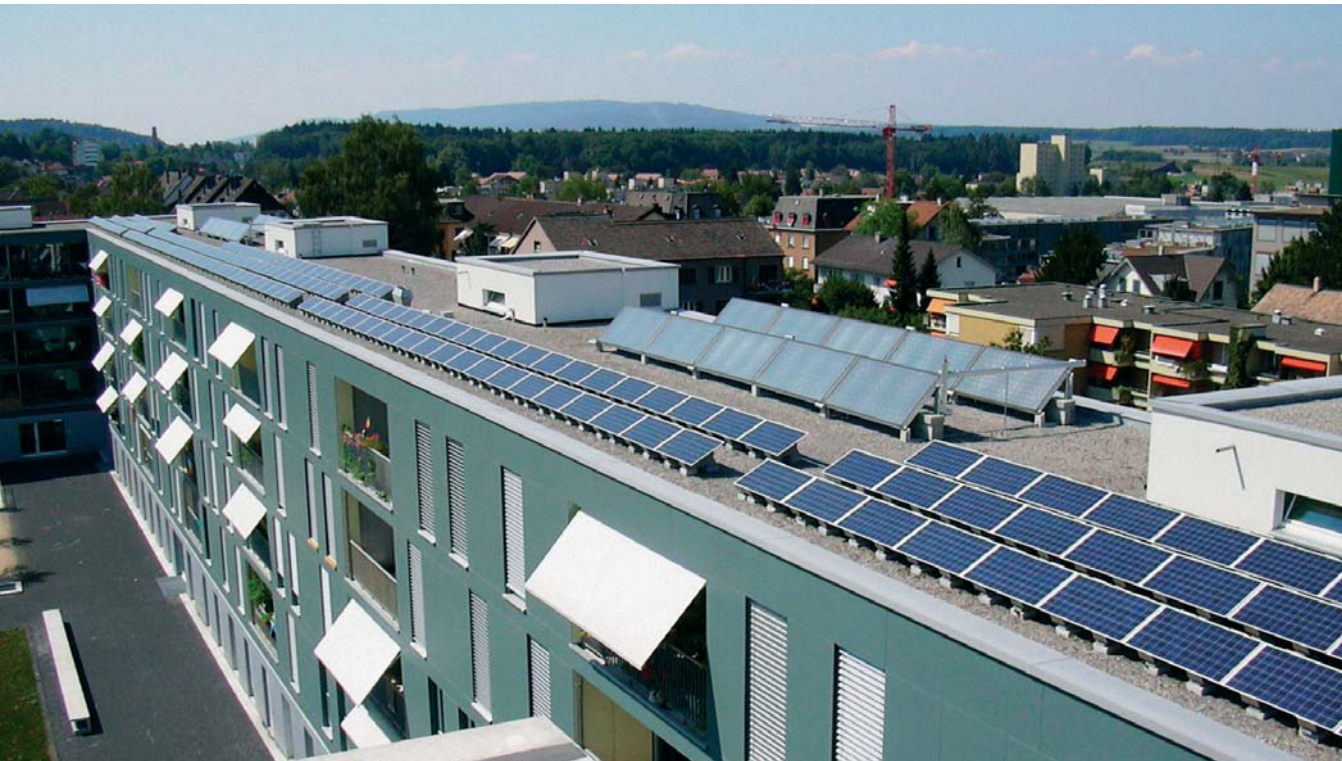
Photovoltaic system Jasminweg in Zürich. The Jasminweg photovoltaic system is operated by Edisun Power AG using plant monitoring services based on satellite information
