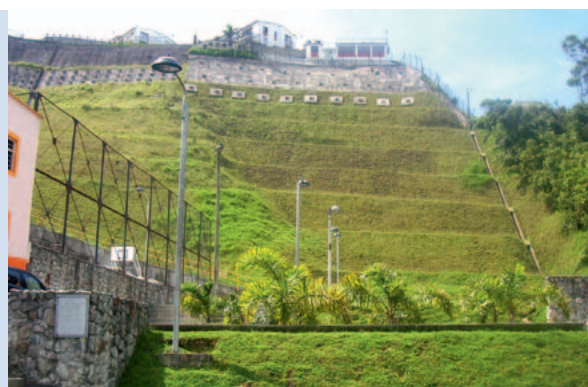
Figure 5: Erosion control and stabilization work in Manizales | Source: Dora C. Suarez
